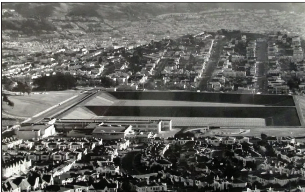
1957 Aerial view of finished reservoir, looking west. Note: Center berm was eventually removed.
